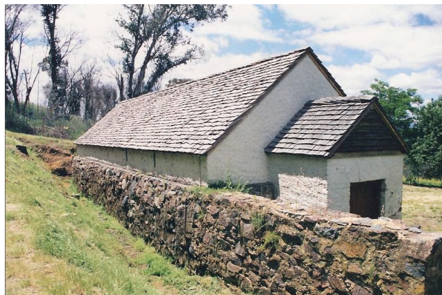
Duntroon Dairy, built c. 18., under threat with inadequate legal protection
